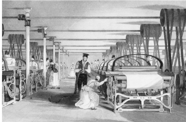
A factory with steam powered looms could produce thousands of times more clothing than traditional “cottage” industry with the same amount of human labor.
